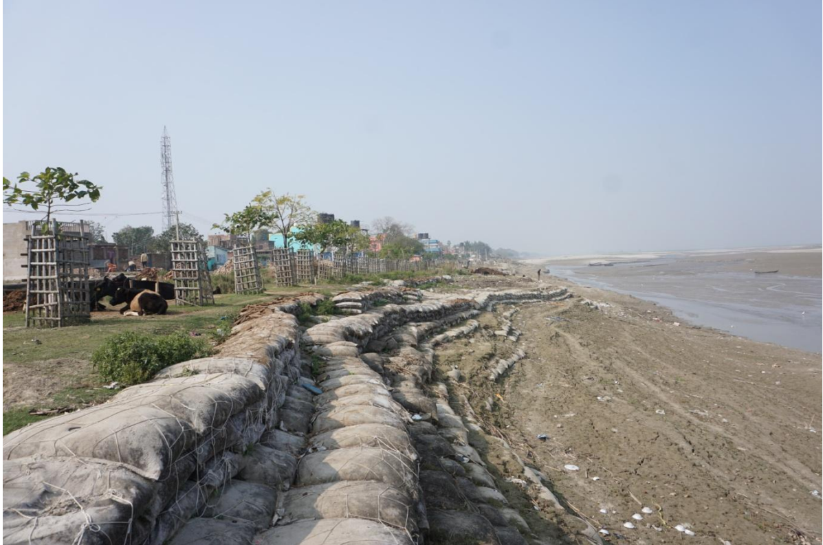
Image 59 : Eroded Bank Stabilied With Geotubes
